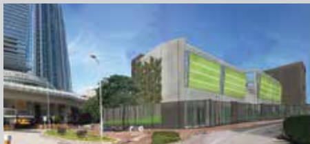
Image courtesy of CLP Power Hong Kong Limited
